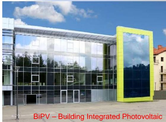
BiPV – Building Integrated Photovoltaic
